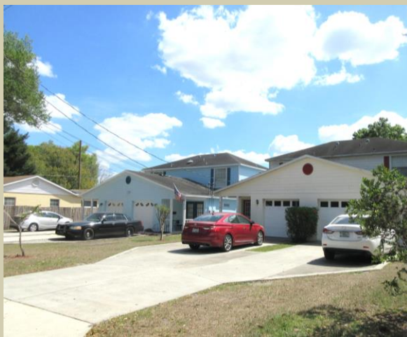
New duplexes on a residential collector street.
