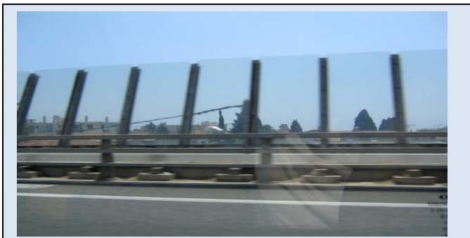
Highway sound walls can take many forms.
