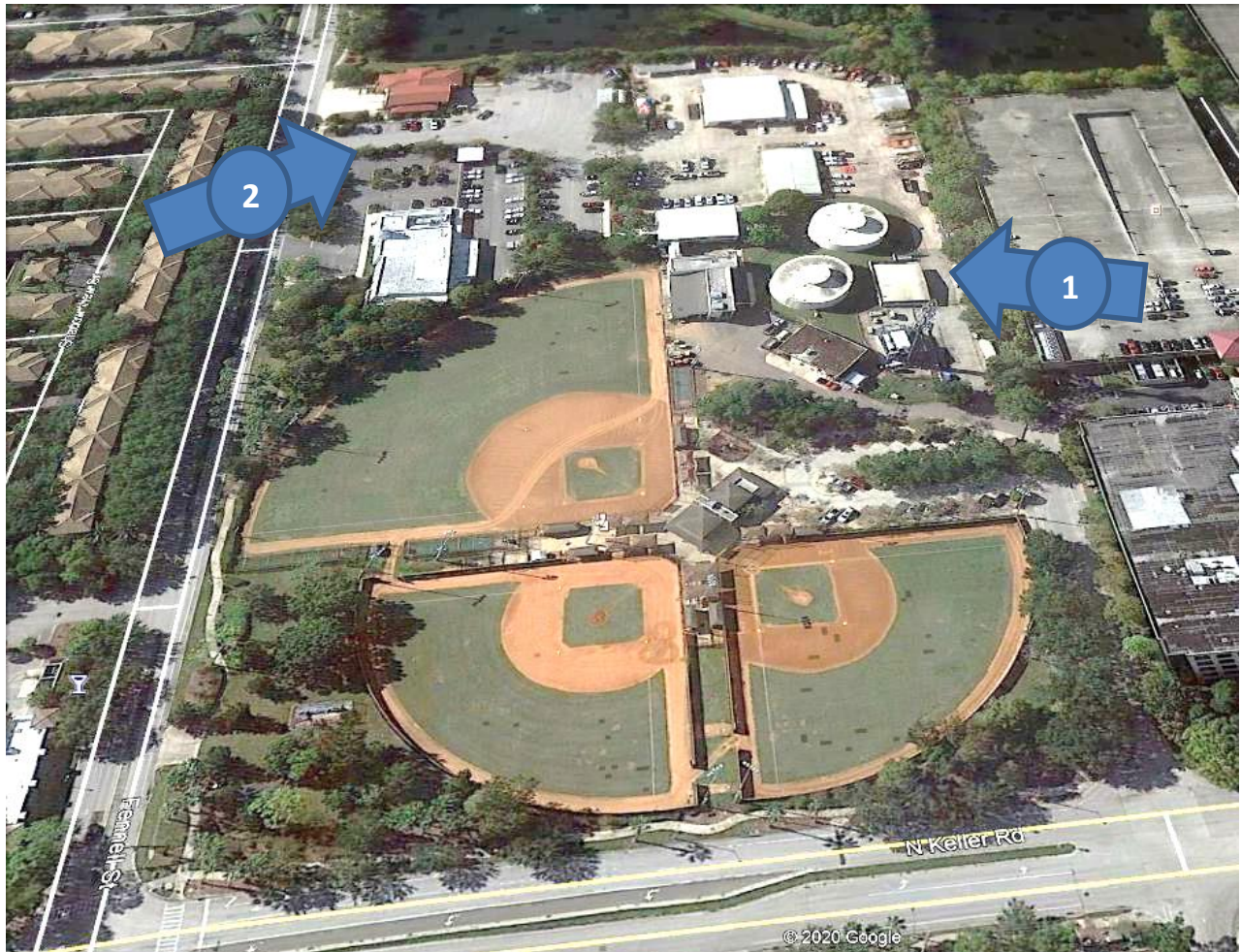
First Station #47 at the top left [1]; public works water plant top right [2] plus ball fields and a concession building. Photo from Google Earth.
